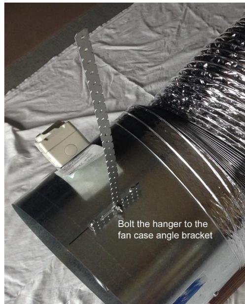
Figure 8. Hanger bracket installation.
