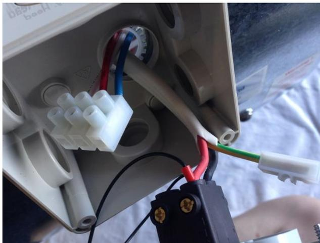
Figure 10. Isolator wiring.
