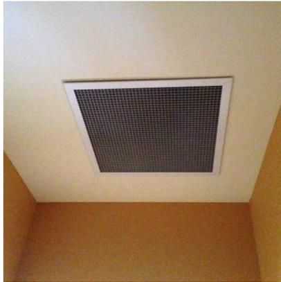
Figure 6. Inlet grill in position.
