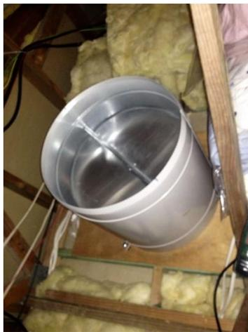
Figure 7. Damper in position.
