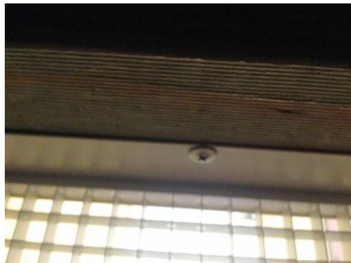
Figure 5. Screw fixing of inlet grill
