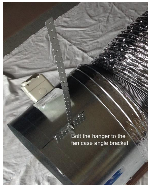
Figure 6. Hanger bracket installation.
