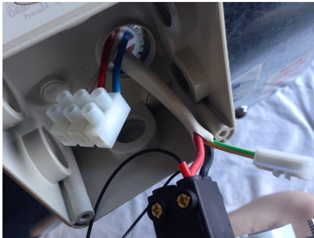
Figure 10. Isolator wiring.
