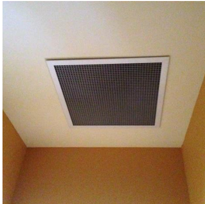
Figure 8. Inlet grill in position.
