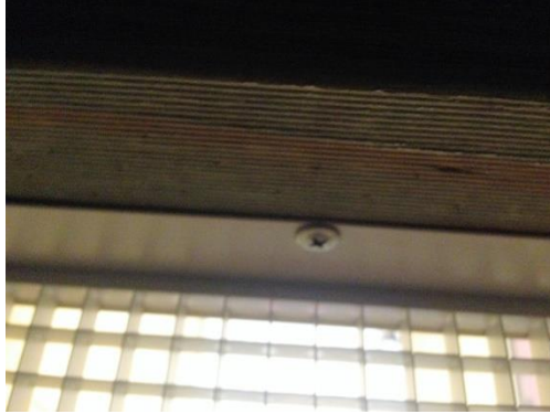
Figure 7. Screw fixing of inlet grill
