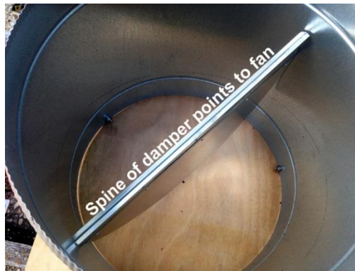
Figure 4. Orientation of damper spine.
